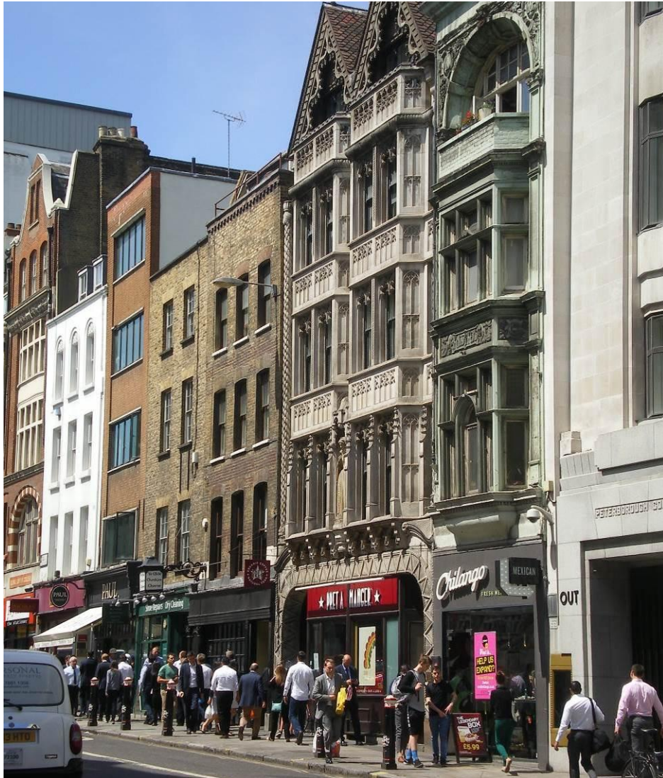
Narrow plots along Fleet Street, ultimately of medieval origin (No. 142-149)
