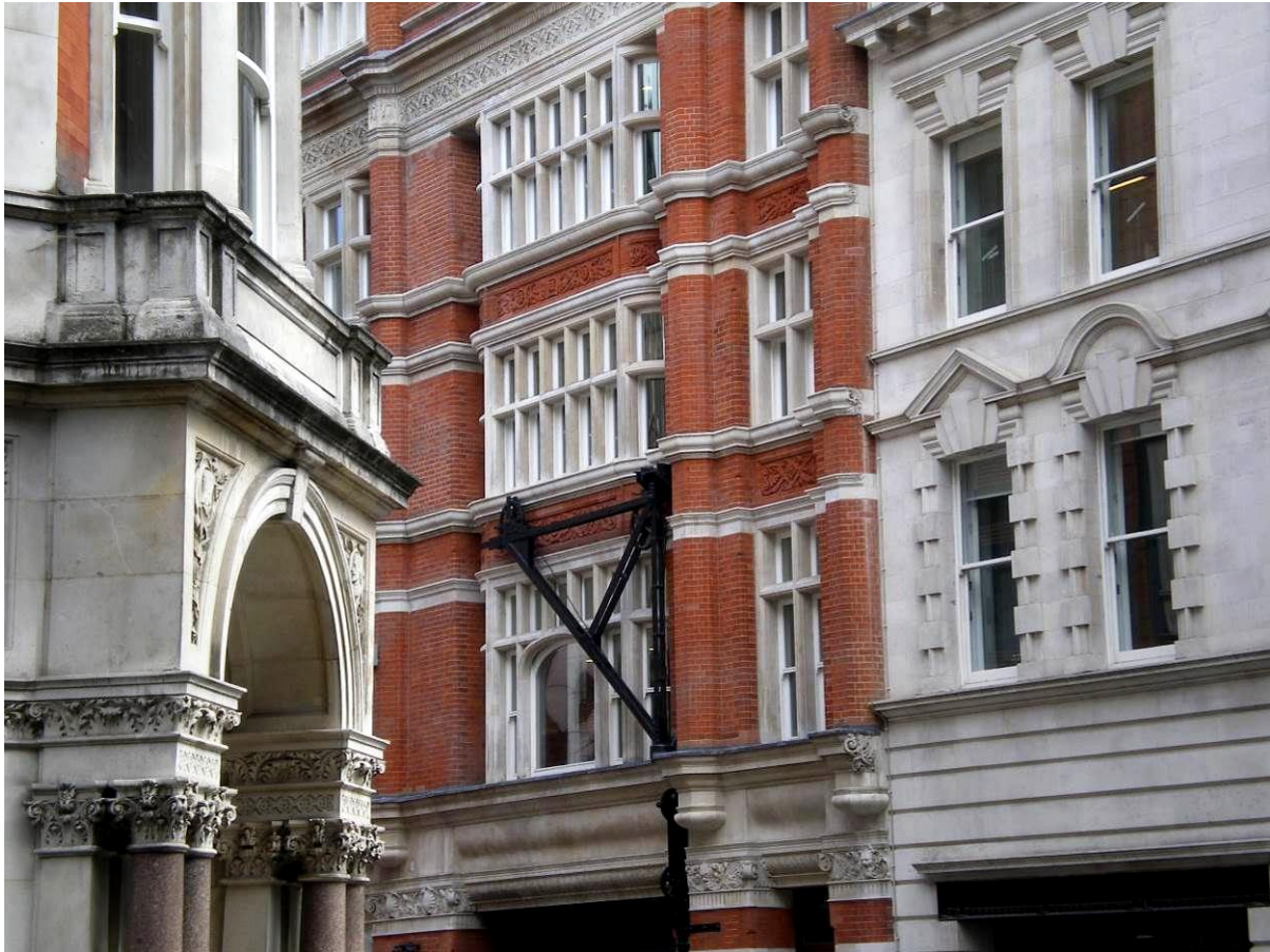
Temple House, Carmelite House and Telephone House (details)
