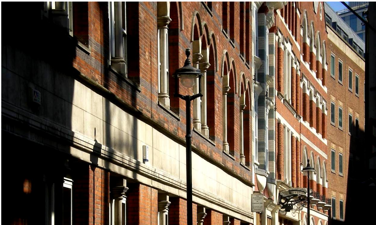
Breams Buildings, North side (detail)
