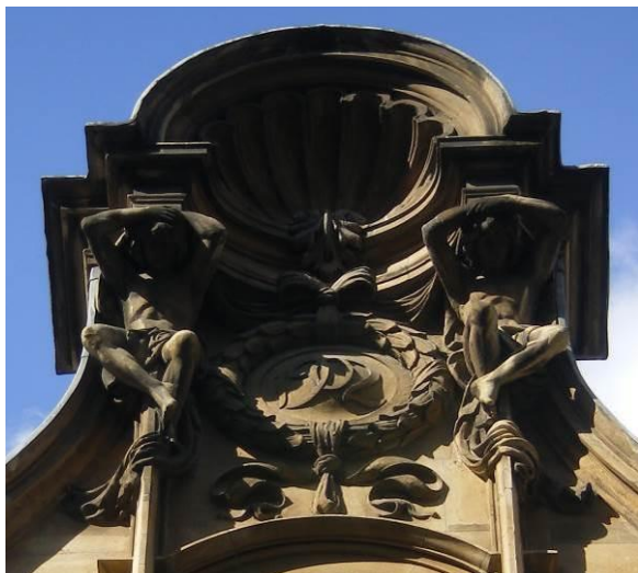
Gable end of No. 78-81 Fetter Lane
