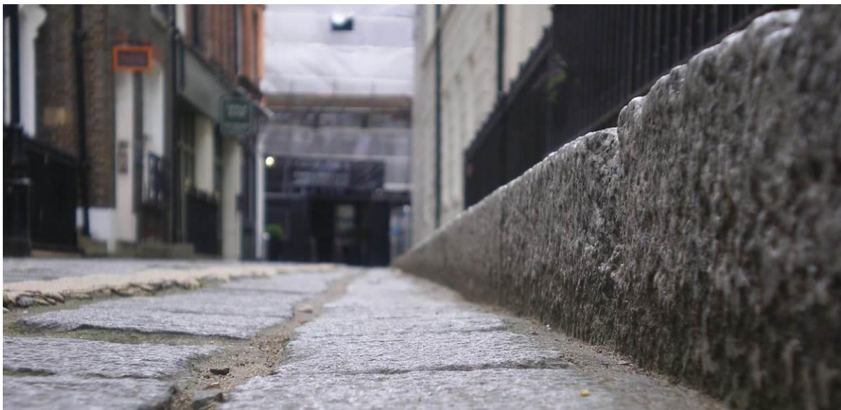
Took's Court, kerb detail
